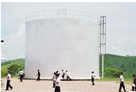
250,000 gallon water storage tank
