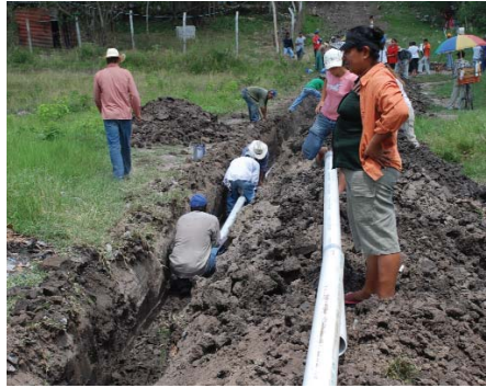
Local laborers installing 4-inch diameter PVC pipe
